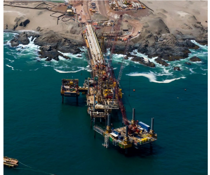
Main jetty at the Port area, September 2022
